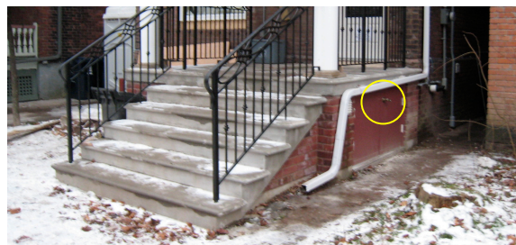
Figure 2. Lockset (circled) to secure under-porch storage
